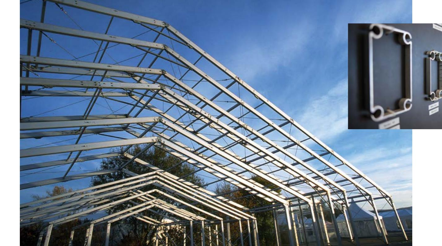
Main elements of RÖDER structures are made of aluminum. Aluminum does not rust; therefore, operating costs are insignificant.
