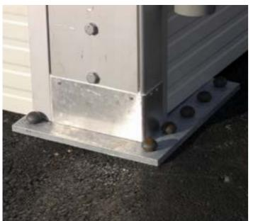
RÖDER solutions are fastened with anchors that do not require a foundation. The unique "heavy floor" technology allows large buildings to be installed without damaging the material. It is possible to assembly a frame tent on any surface.
